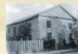
In 1870, the Old African Church was renovated and housed both an elementary school and the first public high school for African Americans in Virginia. Site No. 12 on the Civil Rights in Education Heritage Trail.
